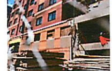
NJ home construction running 45% ahead ...
